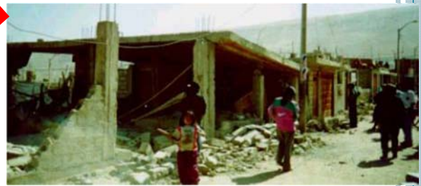
Damage to masonry buildings ( Earthquake 23/06/2001, Magnitude m_v = 6.9 (igp) Magnitude m_s = 7.9 (igp) Epicenter: Front Ocoña )
